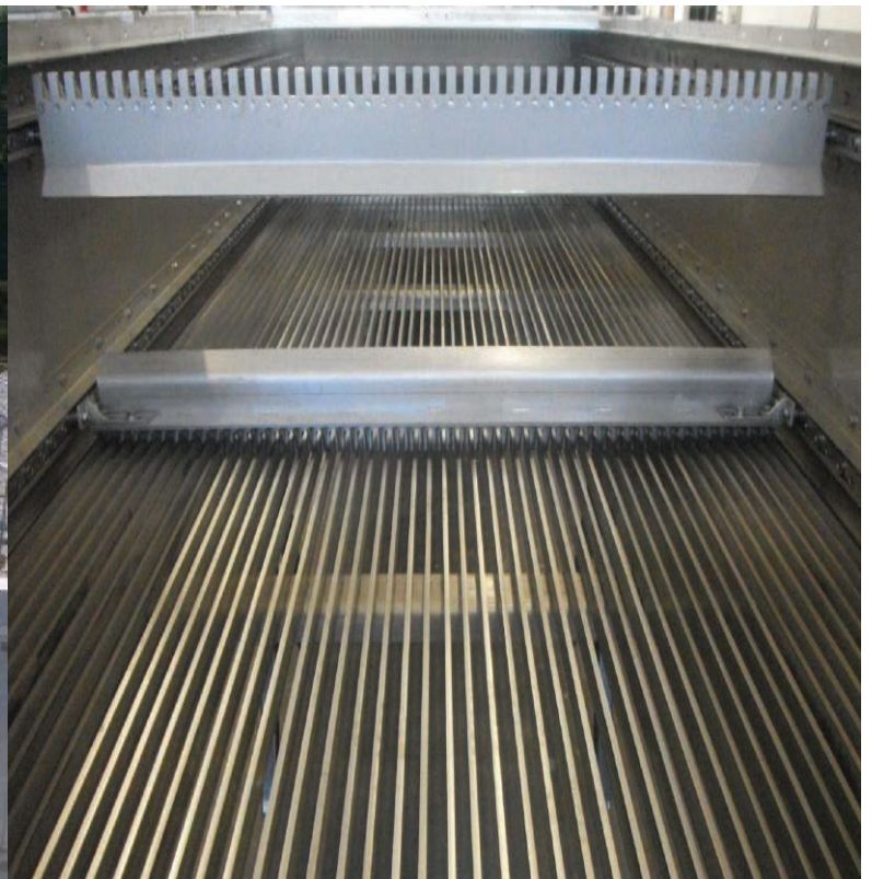
Close-up of bar and rake mechanism from CBS screen
