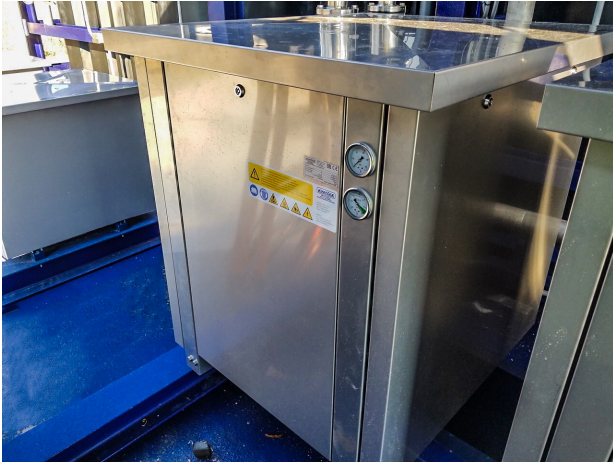
Kubicek PD blowers installed in A3-USA MBR
