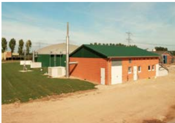
The technical building and the fermenter. It has a net volume of 3,4000 cubic meters.
