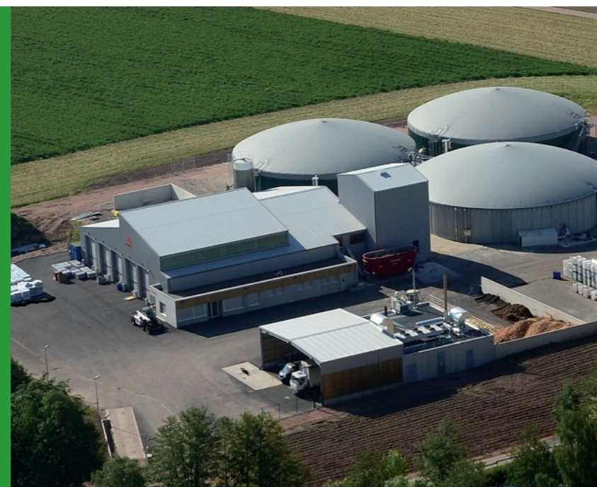
←← In Wales, the food factory Rogerstone Park uses its biogas plant to supply itself with energy.
